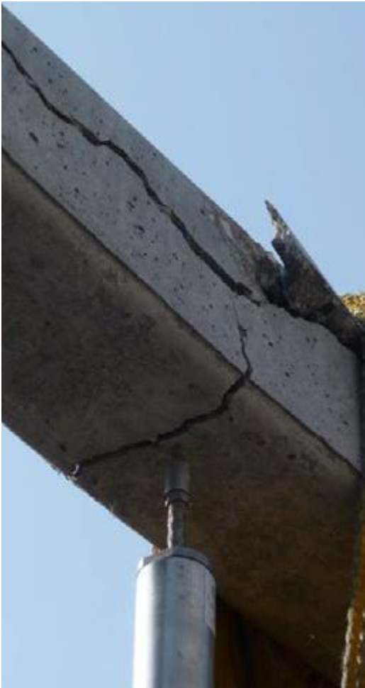
Pole breakage
