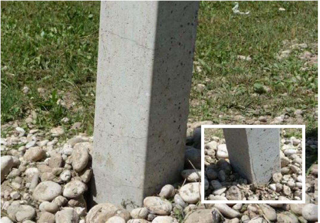
POLE CRACKING
